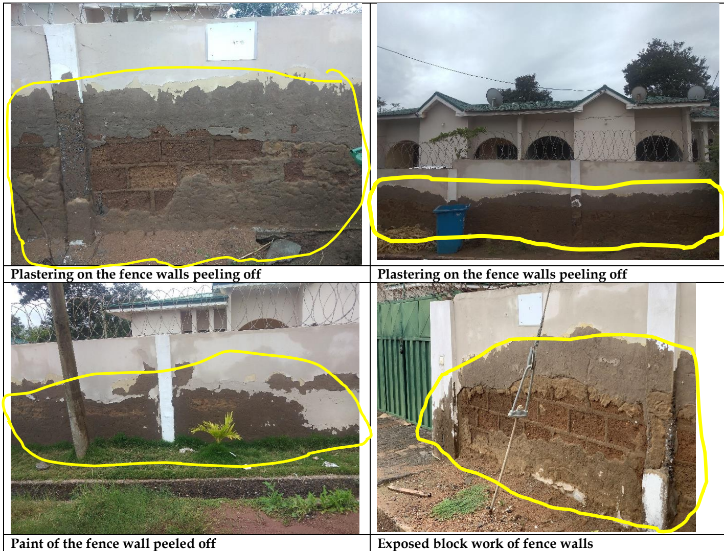
Picture 5: Examples of MRH bungalows that had not been maintained at Spintex, Baatsonaa
