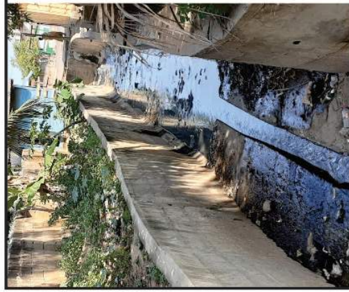
8. 90m x 2.50m x 1.00m rectangular plain concrete drain at Abeka Lapaz (2017). -100% completed
