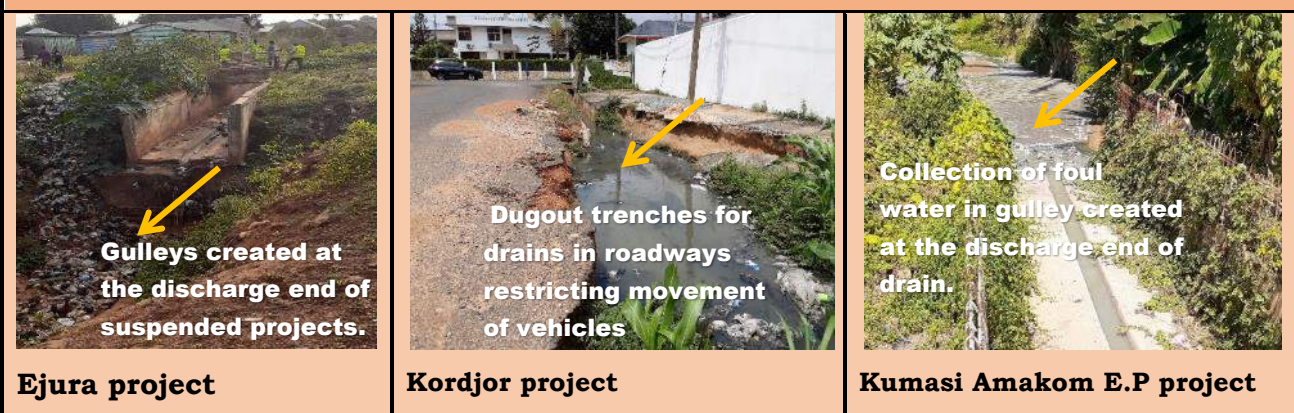
Picture 9: Gulleys and stagnant water created by delayed and stagnated projects.
