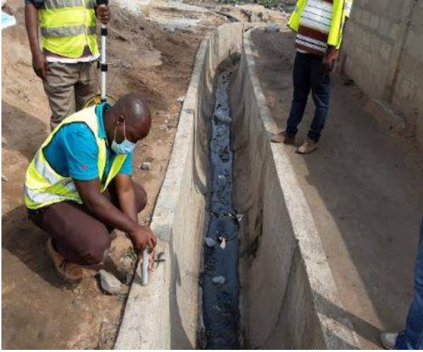
Picture 3: Measuring the concrete strength of a drain (using the Schmidt hammer).
