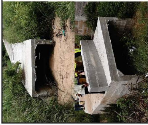
8. 90m x 2.50m x 1.00m rectangular plain concrete drain at Abeka Lapaz (2017). -100% completed
