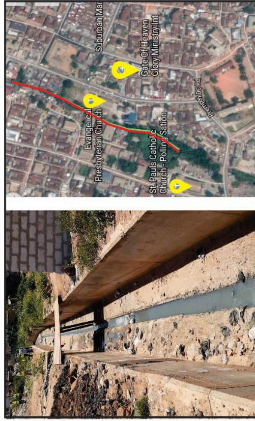
18 165m x 3.5m x 2.00m rein. concrete drain at Kumasi Amakom E.P Church. (Redesigned to 350m x 2m x 2m rein. concrete drain-100% completed)
