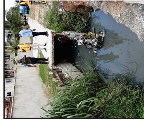
4. 15.00m x 3.50mm x 1.50mm reinforced concrete open drain at Ashiyite. (Redesigned to 16m x 4m x 2m box culvert- 100% completed)
