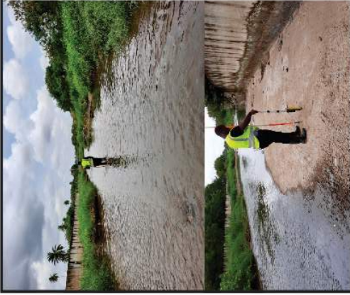
22. 2200m x 25.0m x 2.5m reinforced concrete drain at Akora (Agona Swedru) -40% completed
