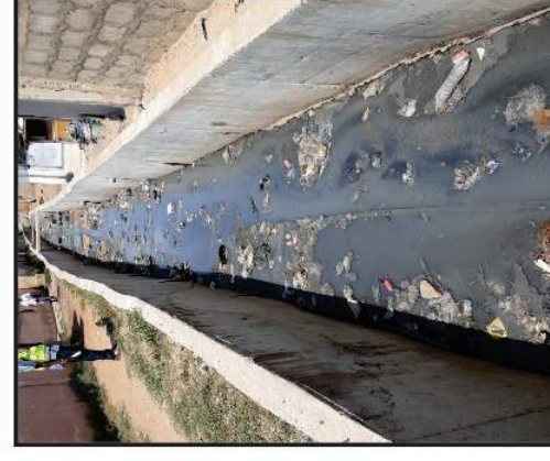
7. 250.0m x 3.50m x 1.50m reinforced concrete open drain at Abeka Lapaz (2018). (Redesigned to 350m x 2.0m x 1.3m rein.conc. drain -100% completed)
