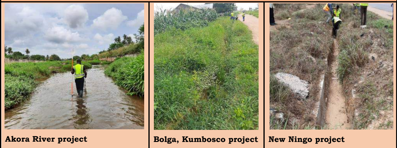
Picture 8: Weed growth in suspended works.
