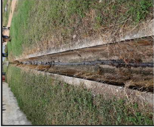
9. 120.0m x 7.00m x 2.50m reinforced concrete open drain at Mallam. (Redesigned to 2no., 23m x 4m x 2.5m and 16m x 9m 2.5m box culverts -52% completed)
