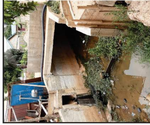
4. 15.00m x 3.50mm x 1.50mm reinforced concrete open drain at Ashiyite. (Redesigned to 16m x 4m x 2m box culvert- 100% completed)
