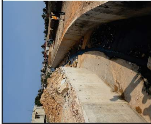
12 250.0m x 3.50m x 1.50m reinforced concrete drain at Nungua. (Redesigned to 250m x 3.0m x 1.8m rein. conc. drain-95% completed)
