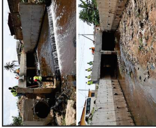
9. 120.0m x 7.00m x 2.50m reinforced concrete open drain at Mallam. (Redesigned to 2no., 23m x 4m x 2.5m and 16m x 9m 2.5m box culverts -52% completed)
