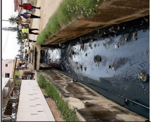
15. 535.0m x 3.50m x 1.60m reinforced concrete drain at Sakaman -100% completed
