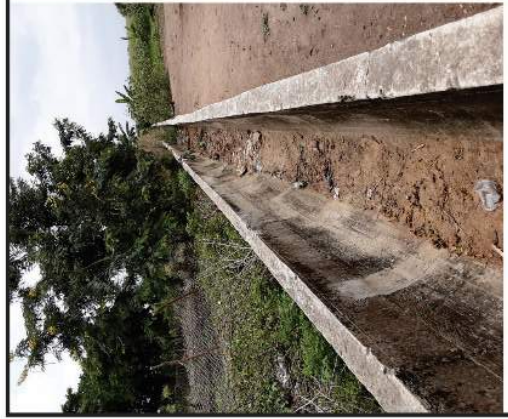
14. 130.0m x 0.90m x 0.90m concrete U-drain at Osuwem- 100% completed
