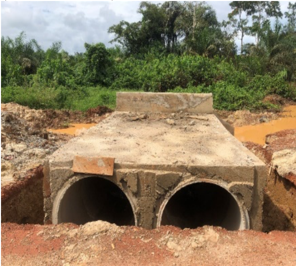
Picture 9: Poor workmanship on 1200mm double pipe culvert on Okumanin -Akokoase - Ofoase Phase 2 (km 16.70 - 32.0) - CRIP Phase II
