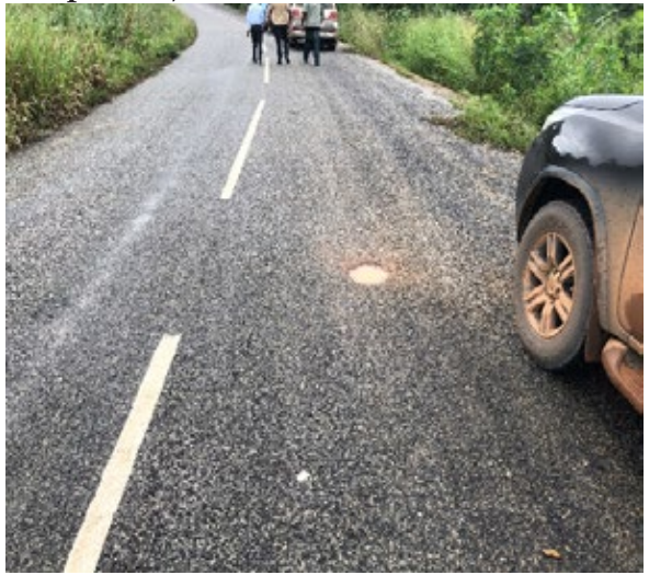
Picture 5: Pothole developing on a section of Kushea - Abotare-Akwawusu-Atweneboana Junction Road from CRIP I completed in 2019 (3 years after completion)
