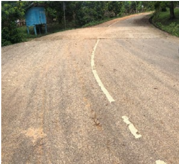
Picture 4: Deterioration at the start of Kushea - Abotare-Akwawusu-Atweneboana Junction road from CRIP I completed in 2019 (3 years after completion)
