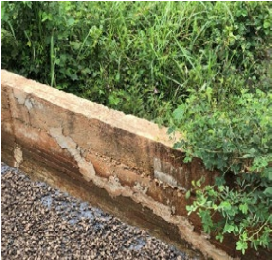
Picture 10: Honeycombs in u-drain patched with mortar at a section of Amantena junction -Wiowso - Senkye road - CRIP Phase II
