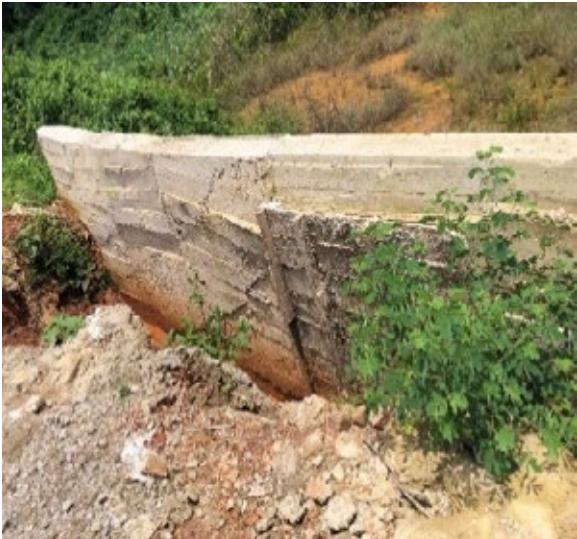
Picture 10: Honeycombs in u-drain patched with mortar at a section of Amantena junction -Wiowso - Senkye road - CRIP Phase II
