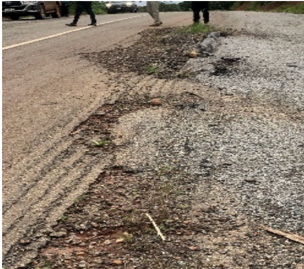
Picture 2: Deteriorated road surface of a section of Dwerebease-Kwahu--Fodoa Ph. II road from CRIP II one year after construction
