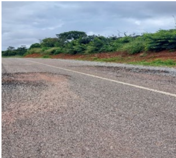
Picture 3: Deteriorated road surface of a section of Dwerebease-Kwahu--Fodoa Ph. II road from CRIP II one year after construction
