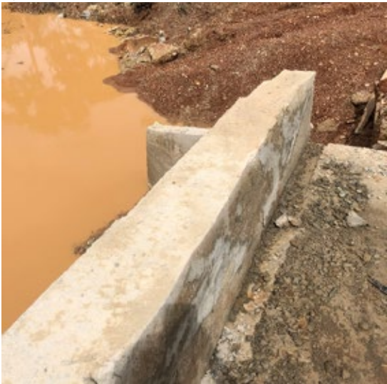
Picture 9: Poor workmanship on 1200mm double pipe culvert on Okumanin -Akokoase - Ofoase Phase 2 (km 16.70 - 32.0) - CRIP Phase II
