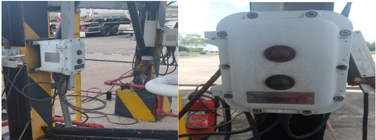
A sample of the old/existing grounding/earthing devices at BOST
