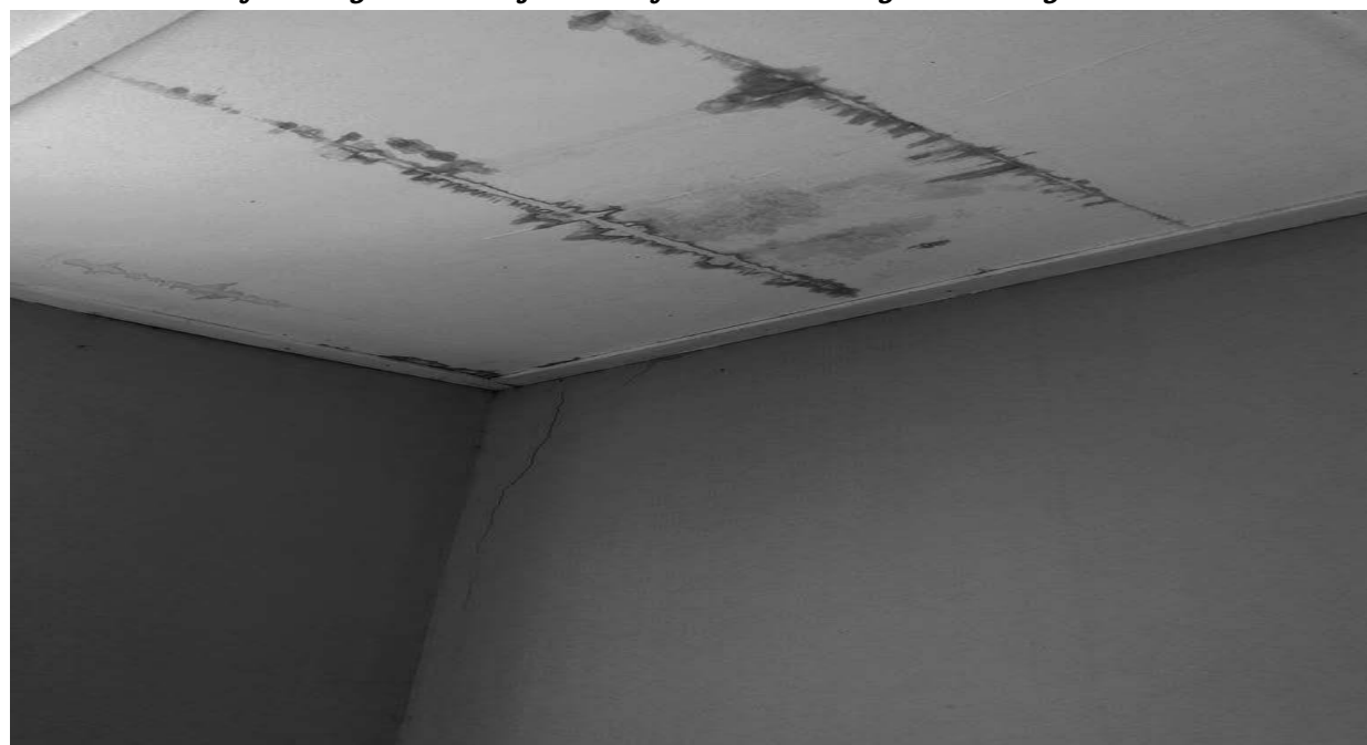
Picture 'A': Roof Leakages on the Ajumako Afranse YLSTI Boys Dormitory
